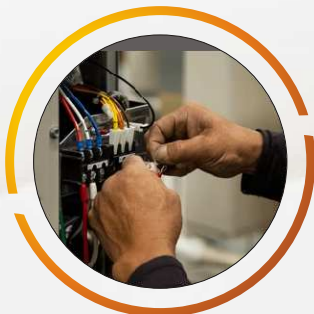
Electrical work HVAC work
